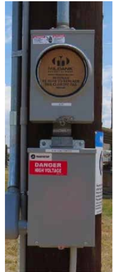
Pole-mount small cell power configuration
